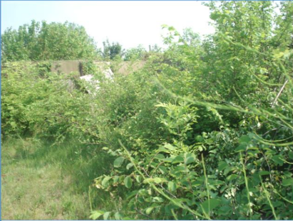
This is a picture of the gun emplacements on the ramparts above the magazine before we went to work on them.
